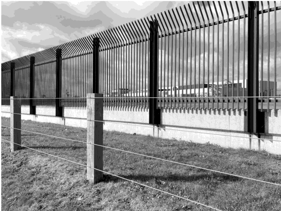
Figure 4 . The wall of the Facebook® datacentre in Odense. Source: Caroline Anna Salling, September 15, 2022.
