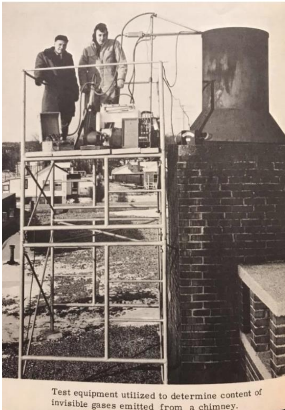
Figure 3 . Test equipment utilized to determine content of invisible gases emitted from a chimney. (Source CTA14 ).
