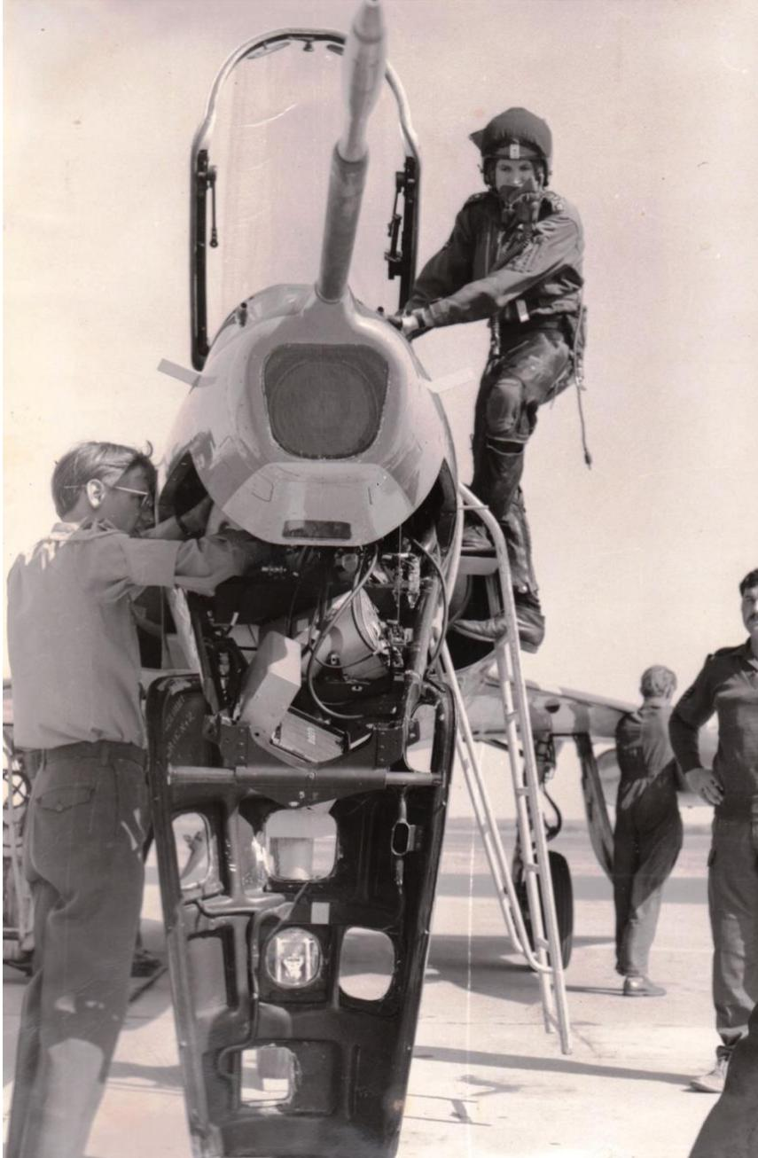
[Figure 3](#). Installation of the camera at the nose of the Mirage, 1976. (Airforce Museum, Cape Town).
